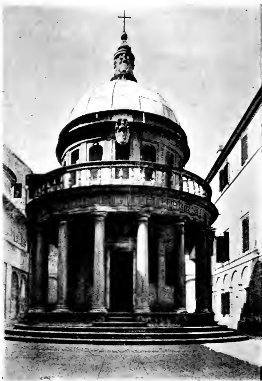
"TEMPIETTO" IN CLOISTERS OF SAN PIETRO IN MONTORIO, ROME. Bramante, Archt.
